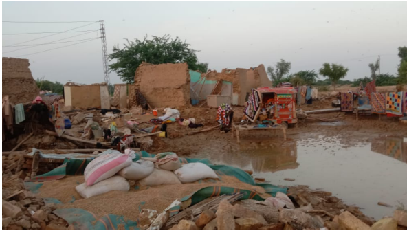
Adobe mud houses partially or totally collapsed
